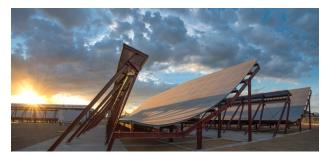
Leolabs has positioned several radars across the globe to track satellites and debris using phased-array technology. Pictured is the Costa Rica Space Radar.
